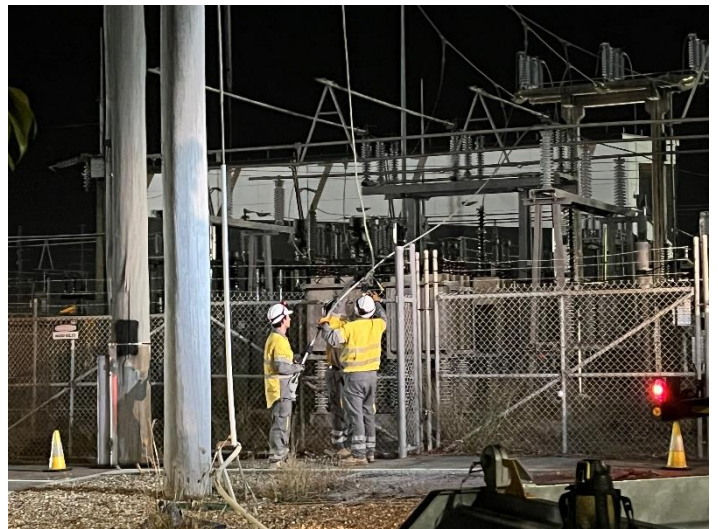
Fig 6 – The powerlines were disconnected from the old substation equipment and removed.
