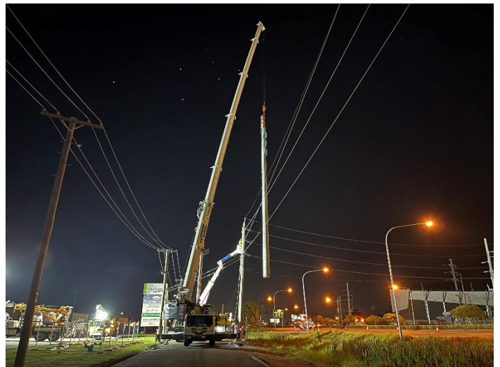
Fig 7 – New concrete pole is craned into position adjacent to Woolcock Street
