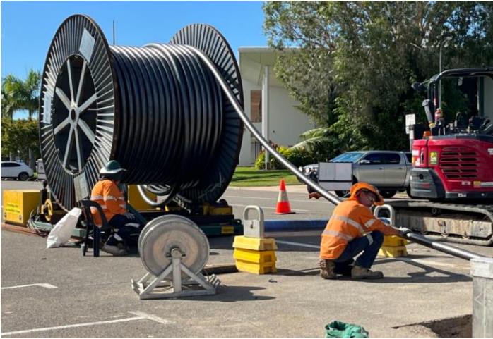
Fig 3 – The exit cables from the Garbutt Substation are joined to the feeder supplying the Belgian Gardens Substation.
