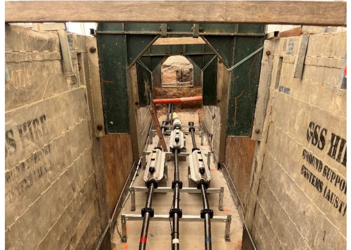
Fig 3 – The exit cables from the Garbutt Substation are joined to the feeder supplying the Belgian Gardens Substation.
