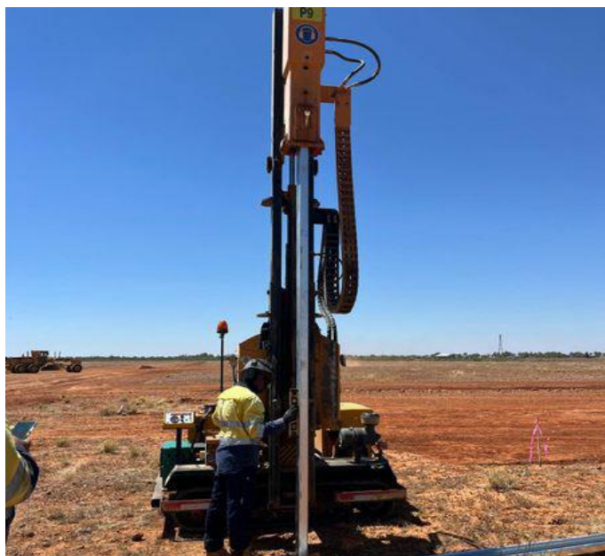
Fig 1 – Pile driver installing the first of the solar array posts.
