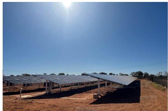
Fig 2 – The first of the solar panels were installed in mid-January.
