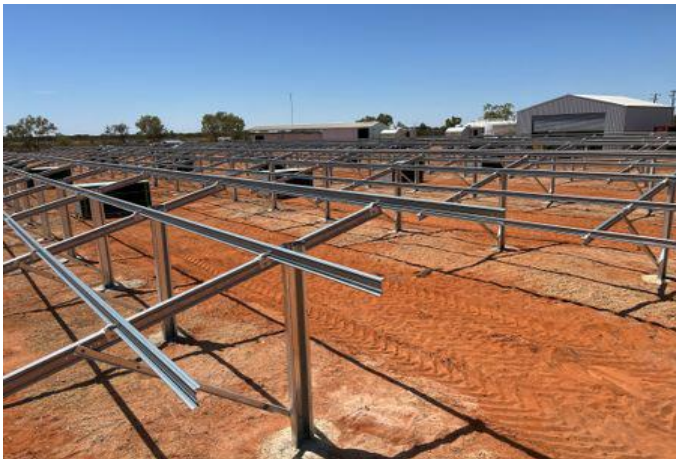
Fig 1 – Installation of the frames for the solar array is well underway.
