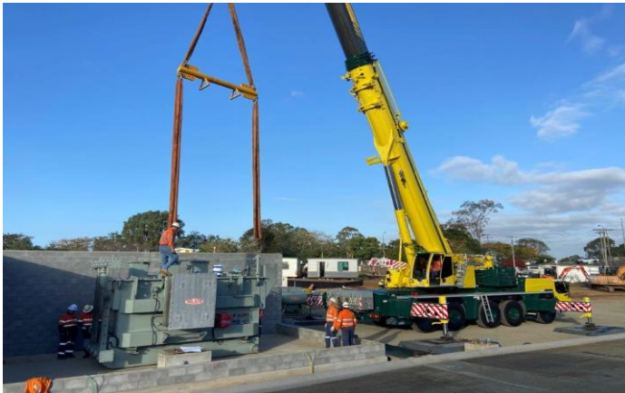
Fig 1 – The transformer is craned into position.
