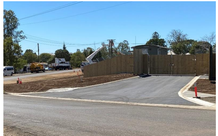
Fig 3 – Crews upgrade the local network around Gracemere.
