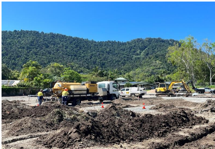
Fig 2 – Contractors excavate trenches for high voltage electrical cables at Cannonvale substation.
