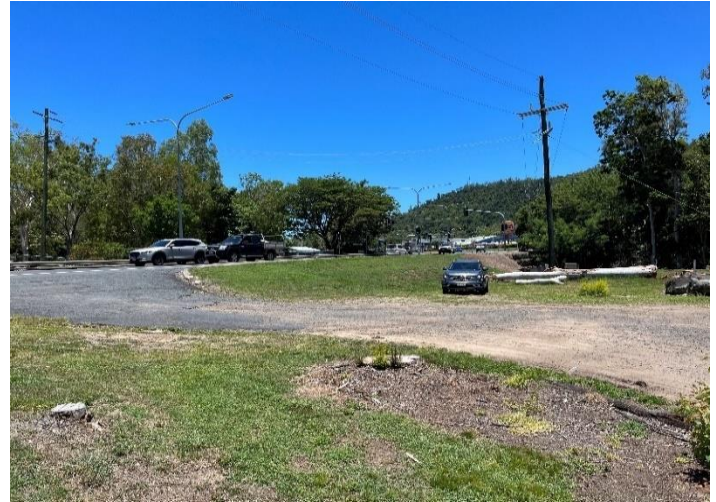
Fig 5 – Access to Cannonvale substation from Shute Harbour Road will be altered to facilitate the delivery of the building.
