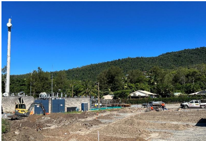
Fig 1 – Civil excavation at Cannonvale substation is underway.
