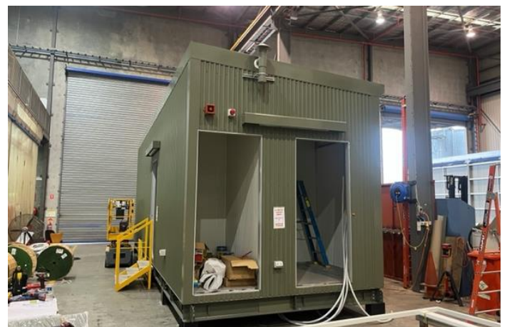
Fig 3 – Fabrication of the modular substation control building is progressing on schedule.
