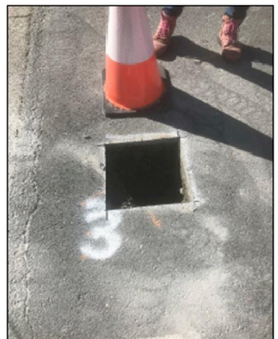
Figure 1 – Hydro excavation access point.
