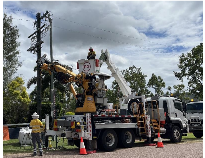
Fig 4 – Townsville's overhead crews dress a new pole ready for a gas switch to be installed at Alligator Creek.
