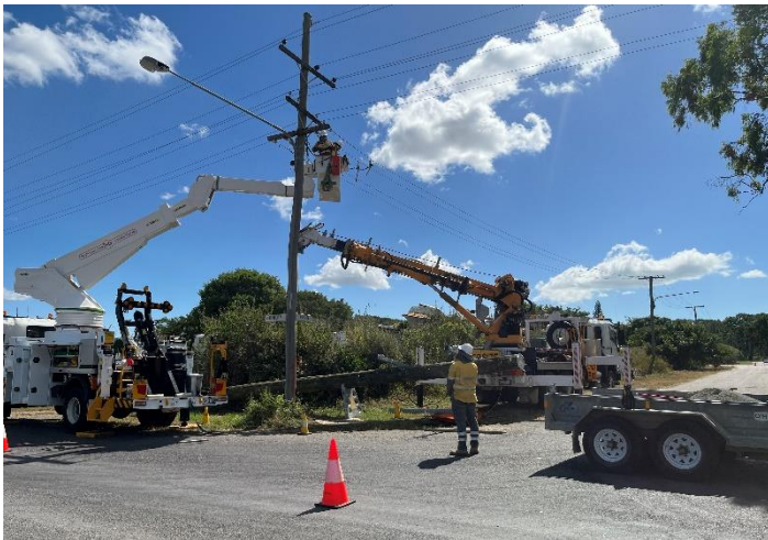
Fig 6 – Local Townsville overhead crews install a new pole and replace poles and crossarms as part of the work to upgrade the local electricity network.
