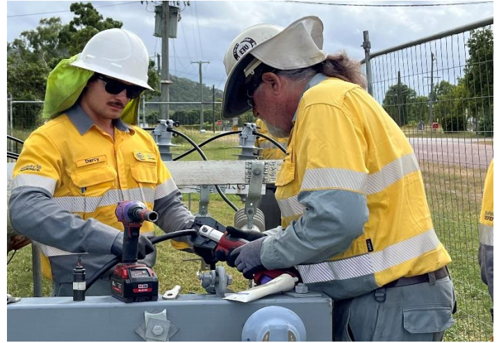
Fig 4 – Townsville's overhead crews dress a new pole ready for a gas switch to be installed at Alligator Creek.
