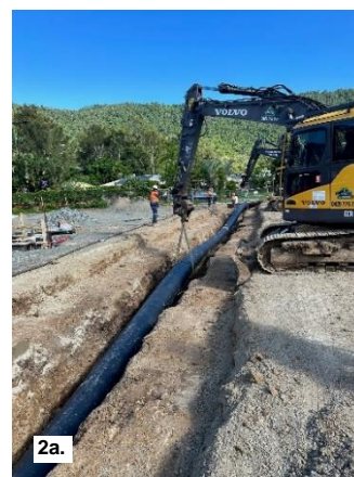
Fig 2a and 2b – The new sewer being line installed with excavator at Cannonvale substation and shoring materials ensure a safe working area in the confined space.
