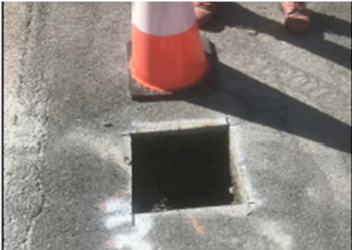
Fig 9 – Hydro excavation access point.
