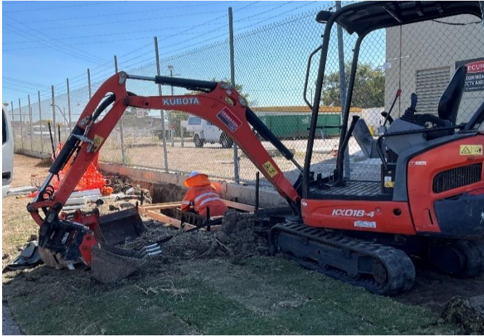
Fig 3 – Installation of the telecommunications pit at the rear of Garbutt substation.
