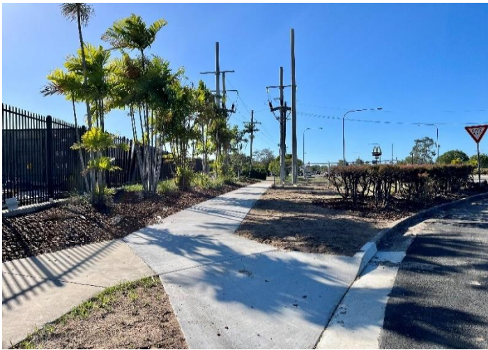
Fig 4 – New footpath installed after civil excavation to install conduit for the 66kV cables.
