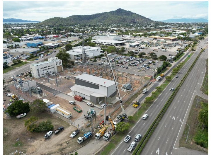
Fig 4 – New footpath installed after civil excavation to install conduit for the 66kV cables.
