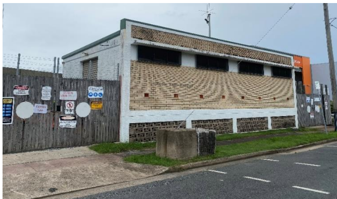
Fig 7 – Tennyson Street substation will be demolished.
