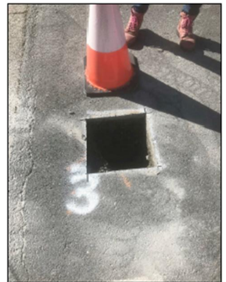
Hydro Excavation Access Point
