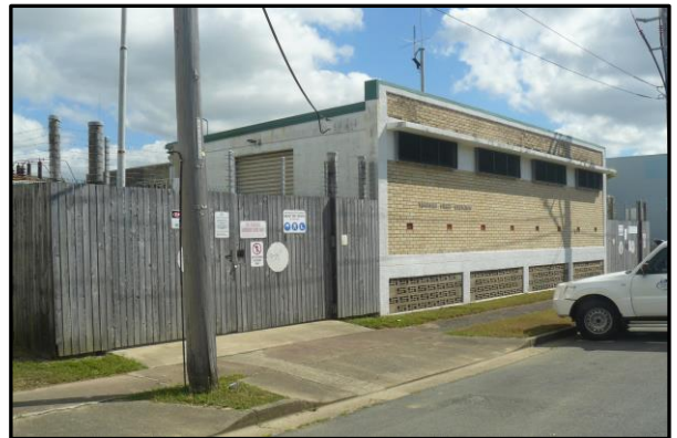
Current Tennyson Street Substation
