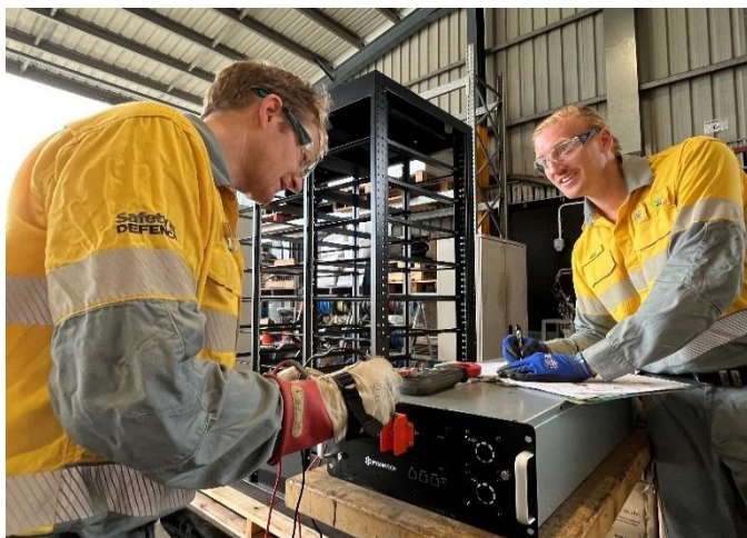
Fig 3 – Testing a battery unit before installing it in the battery rack.
