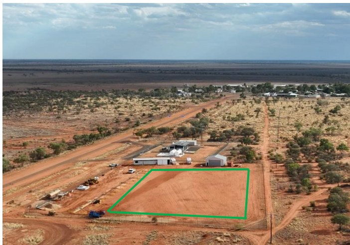
Fig 3 – The location where the new solar array is being constructed.
