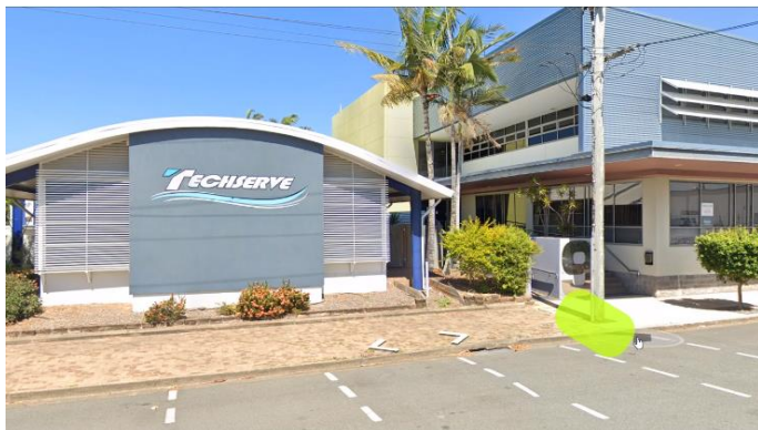
Fig 10 – Location of excavation to access Victoria Street cable in footpath
