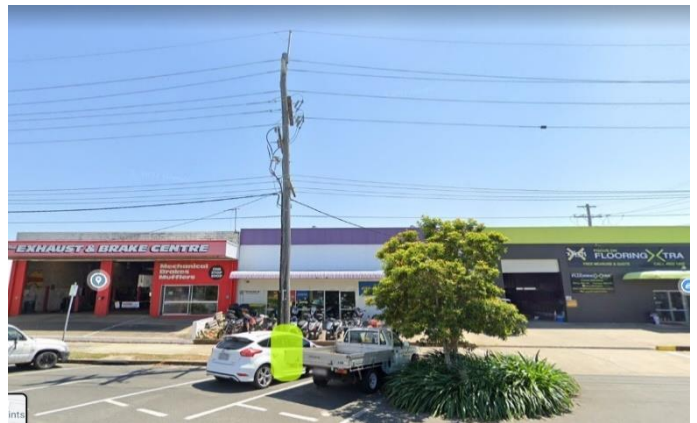
Fig 12 – Location of excavation to access Brisbane Street cable in footpath
