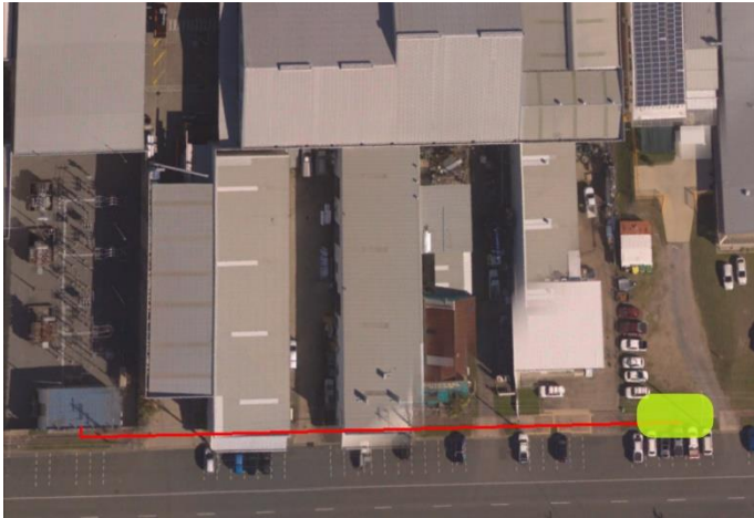
Fig 2 – The first location for civil works excavation to access the old Centrepoint cable.
