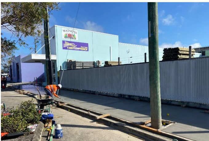
Fig 5 – The contractor's level and compact the new slab in Gordon Street.
