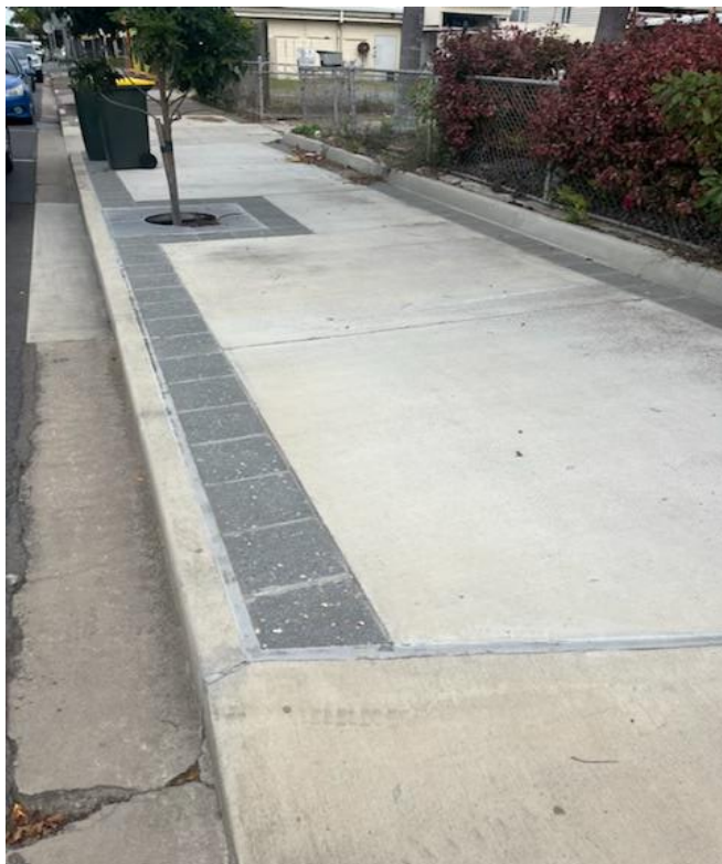
Fig 1 – Example of what the footpaths will look like once reinstated.
