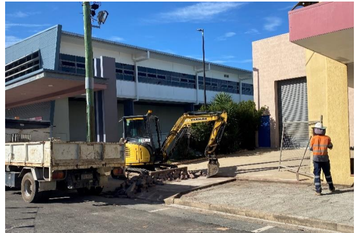
Fig 6 – Contractor's progress the excavation of the footpath down Tennyson Street.
