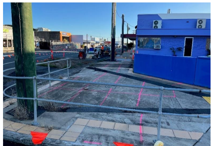
Fig 2 – Footpaths marked up for saw cutting the concrete footpath.
