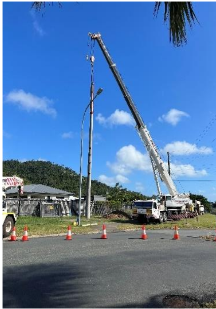
Fig 10 – concrete pole at Jubilee Pocket is craned into place.
