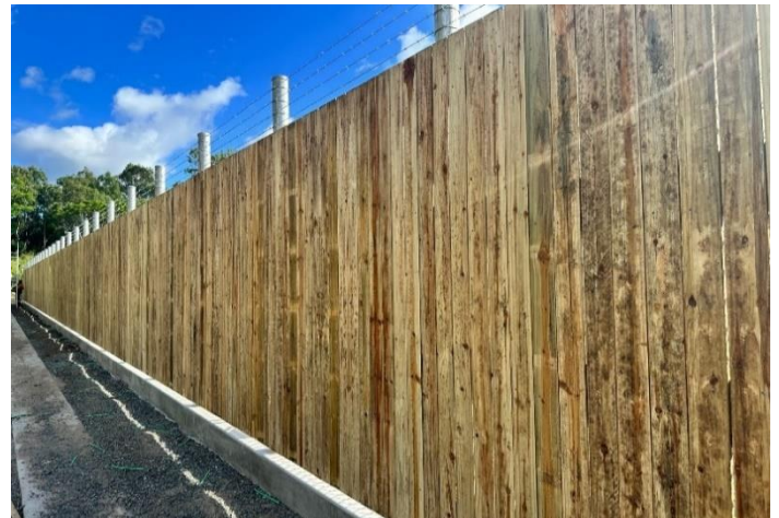
Fig 2 – Perimeter security fencing around the substation is complete.
