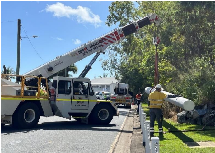
Fig 7 – concrete poles delivered to site on Shingley Drive.
