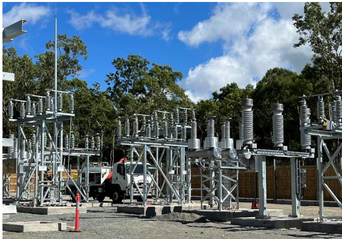
Fig 1 – steelwork in the outdoor switch yard being constructed.
