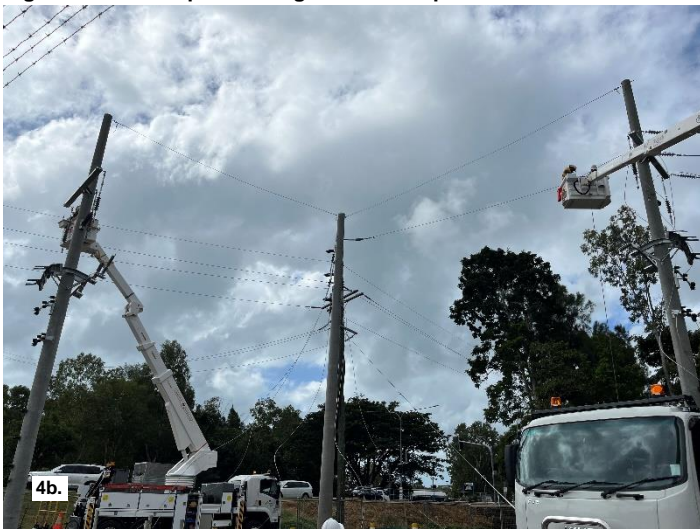
Fig 4b – Ergon crews connecting powerlines to the new poles.
