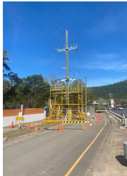
Fig 9 – An example of scaffolding erected for cable termination work.
