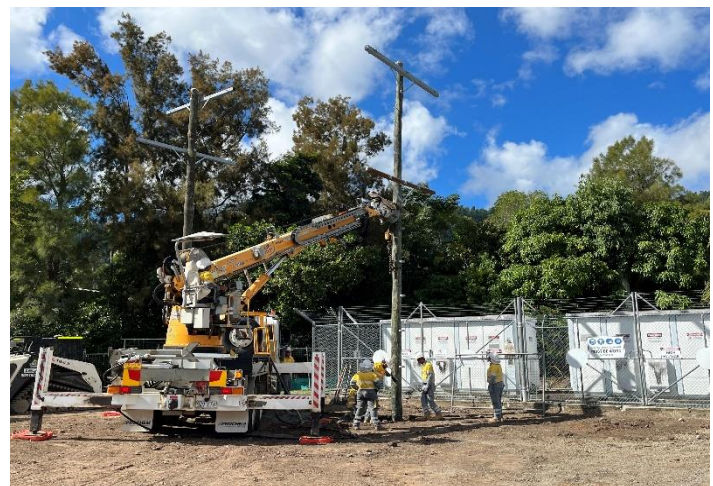
Fig 3 – Poles being installed for network generation at Cannonvale substation.
