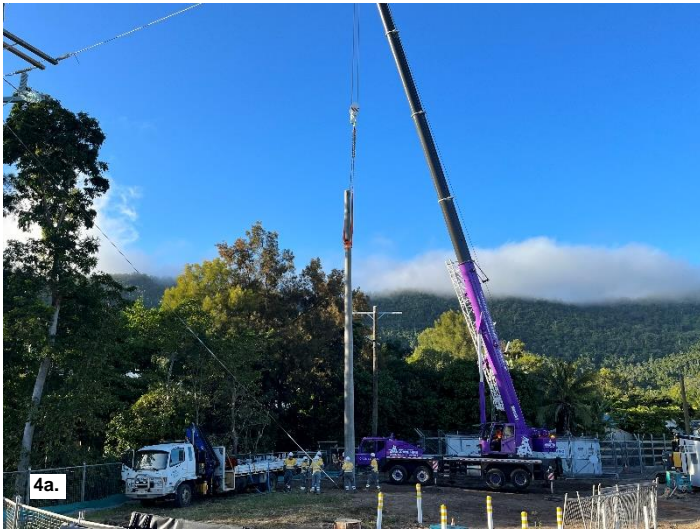
Fig 4a – Concrete poles being craned into position
