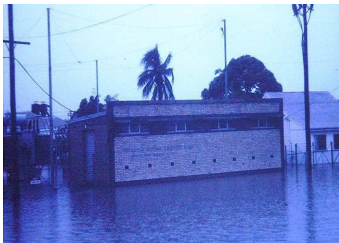
Fig 1 – Tennyson Street Substation inundated in 1974 floods
