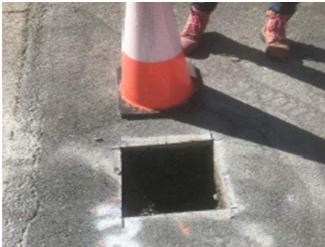
Fig 3 – Hydro Excavation Access Point
