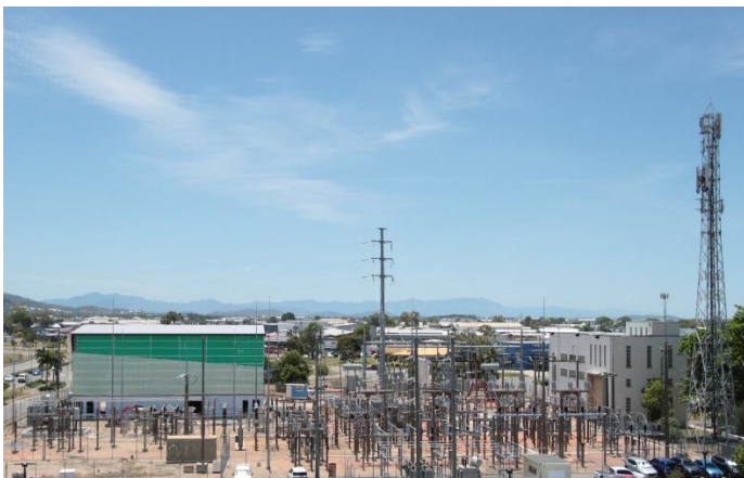
Figure 1 – New Garbutt substation building under construction
