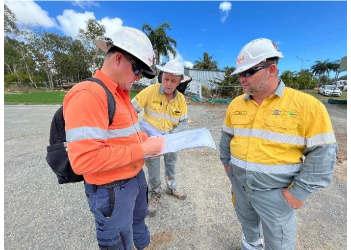
Fig 5 – Ergon staff and Universal Cranes representative plan the delivery and installation of the substation new control building.
