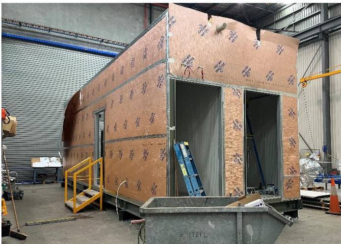
Fig 4 – Fabrication of the modular substation control building has commenced.
