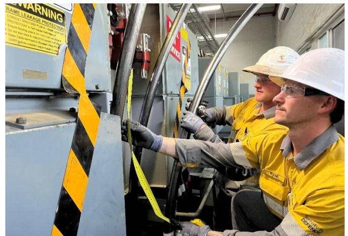
Fig 2 - The underground crew connecting the cables in Stuart substation.
