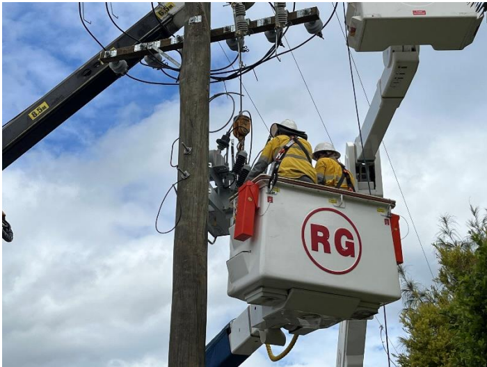
Fig 3 - Local overhead crew installing a new gas switch at Alligator Creek
