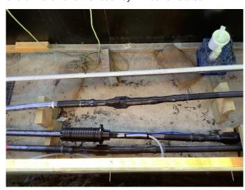
Fig 2 – Cables from the surrounding electricity network are connected to cables from the new substation.
