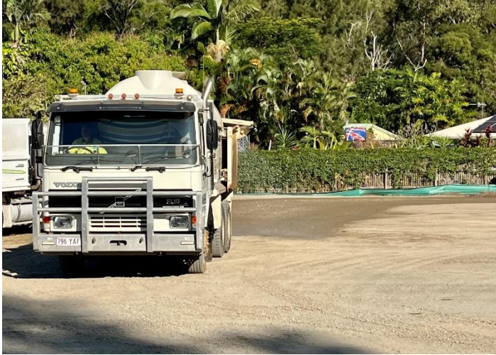
Fig 3 – Water trucks dampen the worksite to mitigate dust
