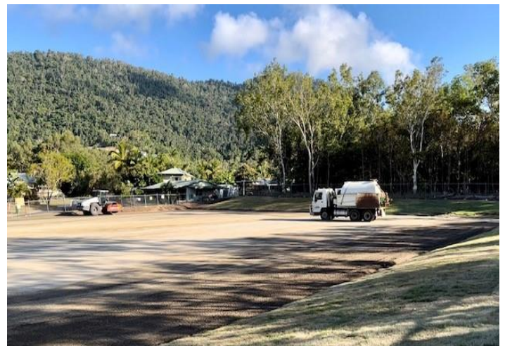
Fig 6 – The site is ready for stage 2 construction work to begin.
