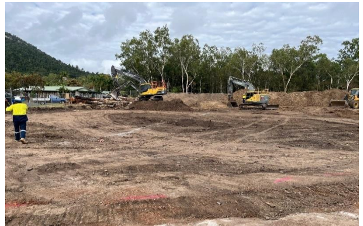
Fig 1 – Early civil works to level substation yard extension.
