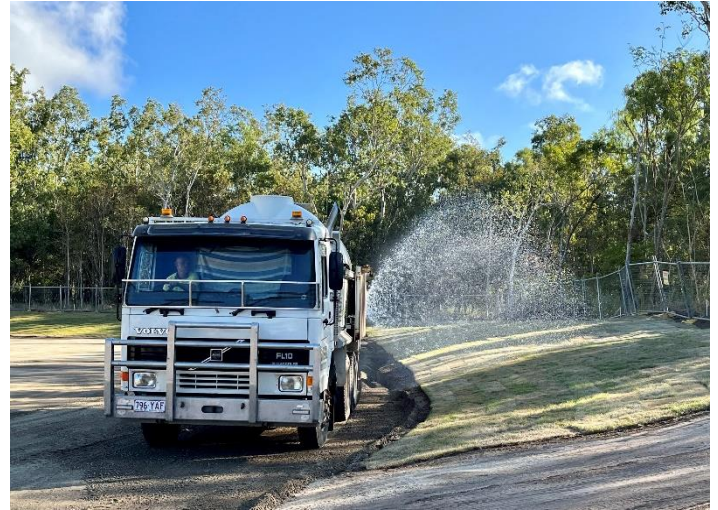
Fig 5 – The area around the slab is turfed to mitigate dust and erosion.
