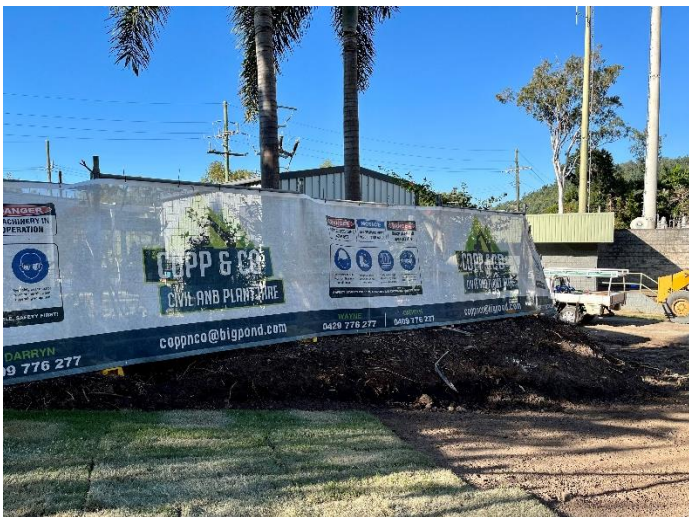
Fig 4 – Fabric material on construction fencing helps to mitigate dust and noise.
