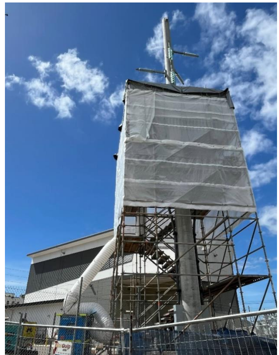
Fig 10 – Scaffolding around a pole for 66kV cable termination works.
