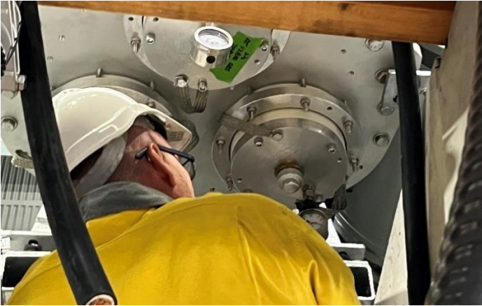
Fig 6 – Ready to degas the GIS pot.
