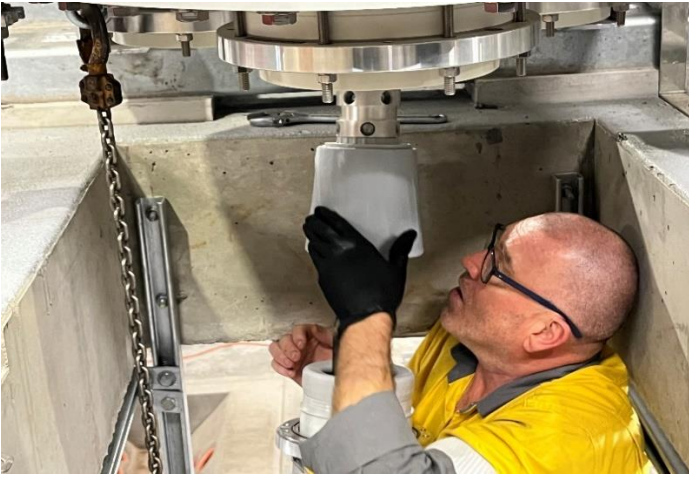
Fig 7 – Termination positioned below the GIS, cleaned, and greased.
