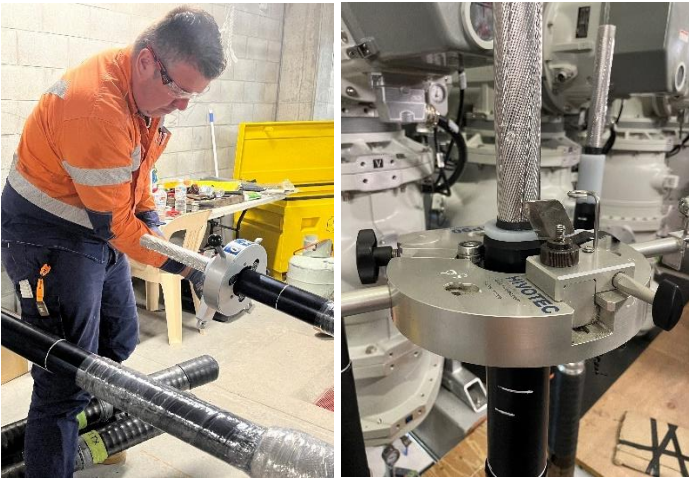
Fig 3 – The insulation is stripped back to reveal the cable.
