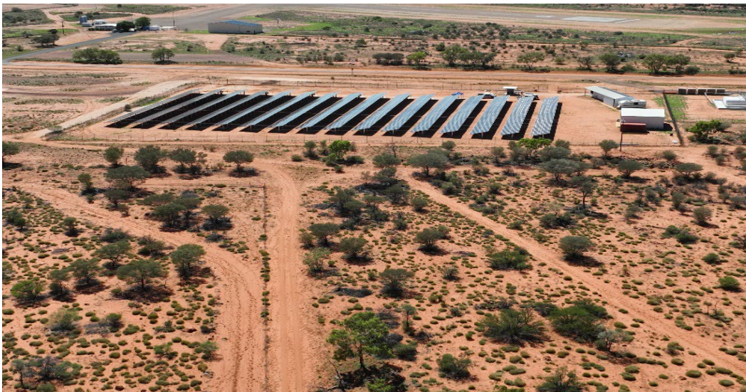
Fig 2- Aerial view of the solar panels
