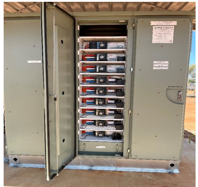
Fig 1-Completed Inverter Switchboard
