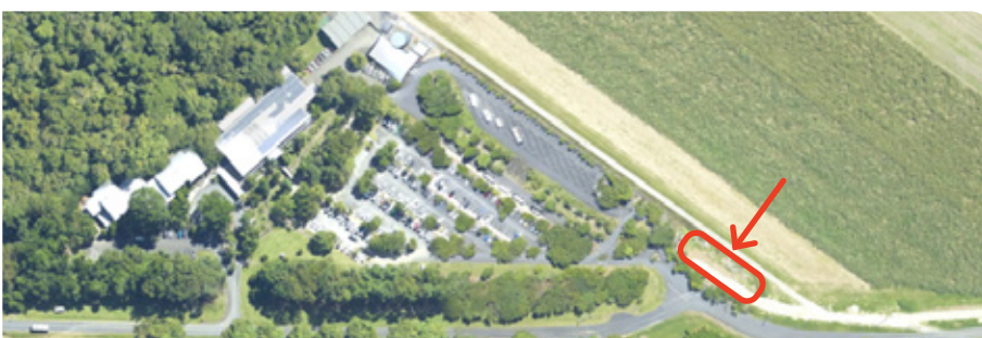
Location of the Mossman Gorge Microgrid adjacent to the Cultural Centre.
