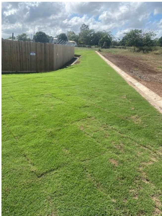
Fig 1 – New turf around the Gracemere substation.
