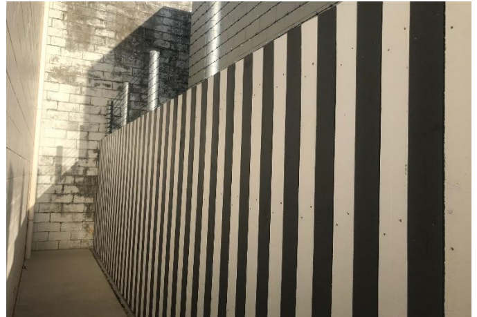
Fig 5 – Completed southern substation security fence.
