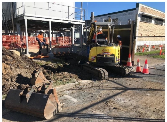
Fig 6 – Stage 1 civil excavation work commences at substation.
