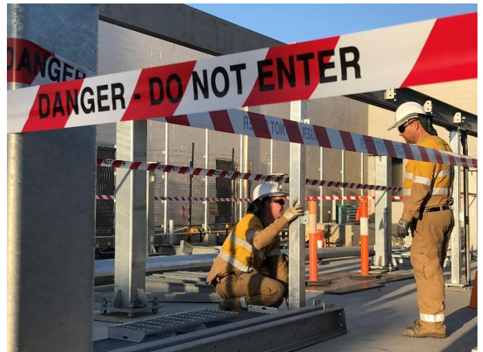
Fig 2 - Crews establish the steel foundations for the buildings.
