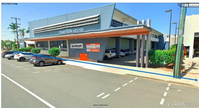
Fig 8 – Location of Victoria Street Feeder civil works.
