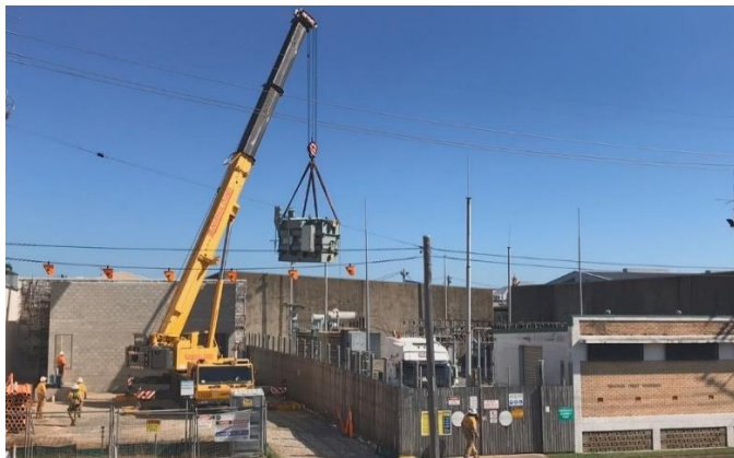
Fig 1 - Transformer No 1 is lifted into place in the new substation.
