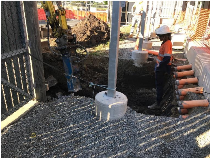
Fig 7 – Excavating the exit cable pit.
